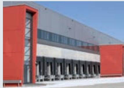
Immogate Logistikcenter, München
